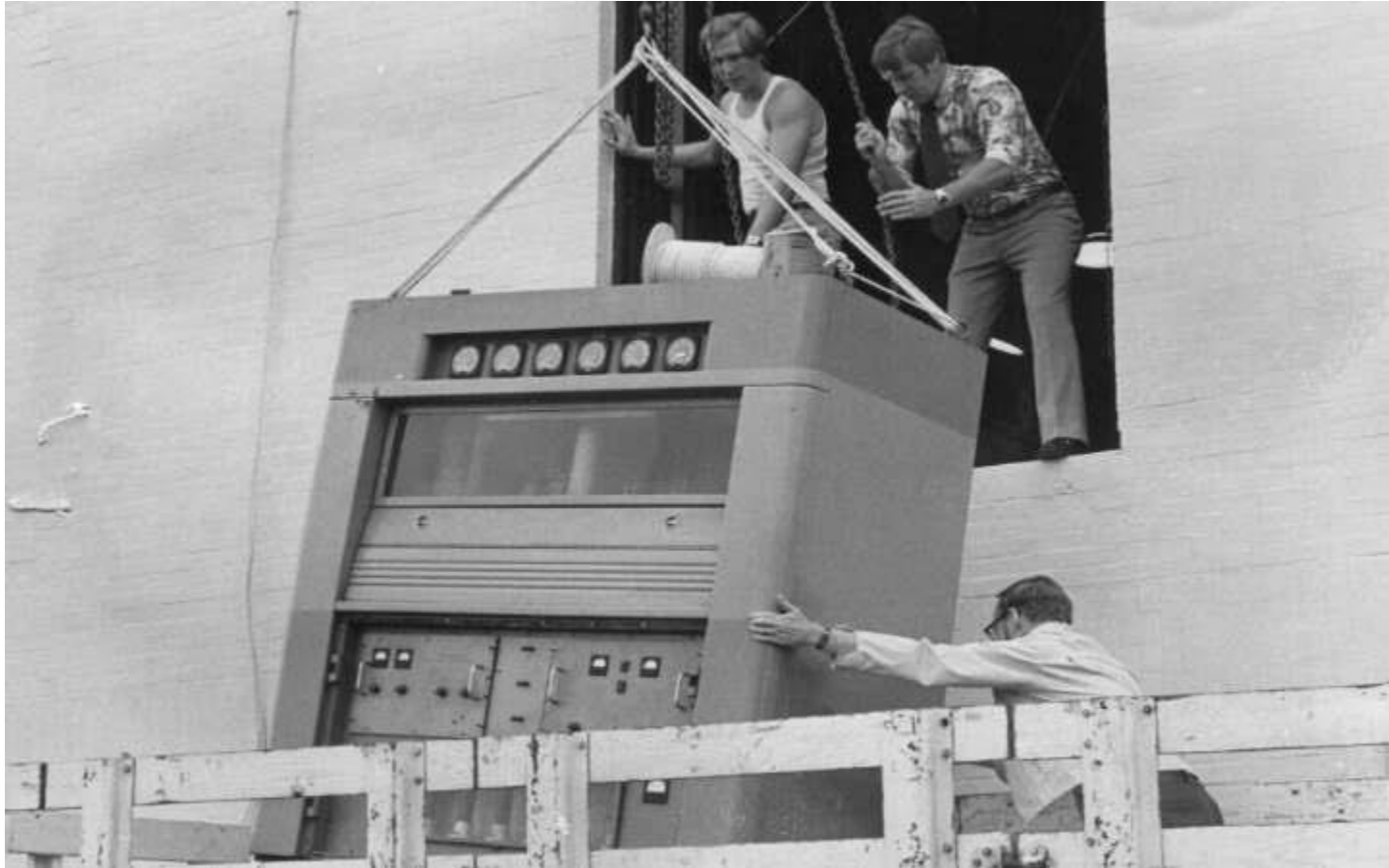
WERG in the 1970's: "new" transmitter being installed in the Nash Library
